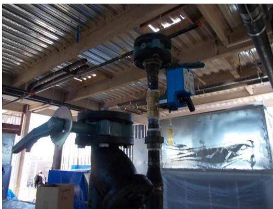
Protect open valve flanges
