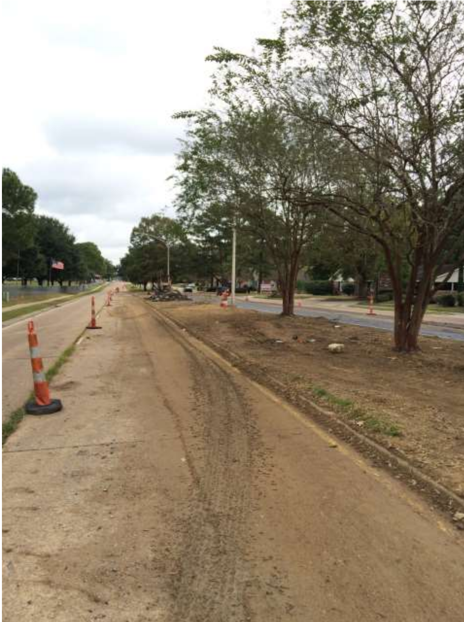
Looking east at the Goodwood Boulevard Median work.
