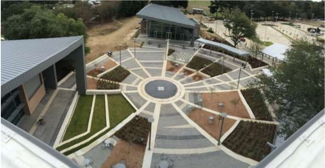
Looking from the roof to the Plaza.
