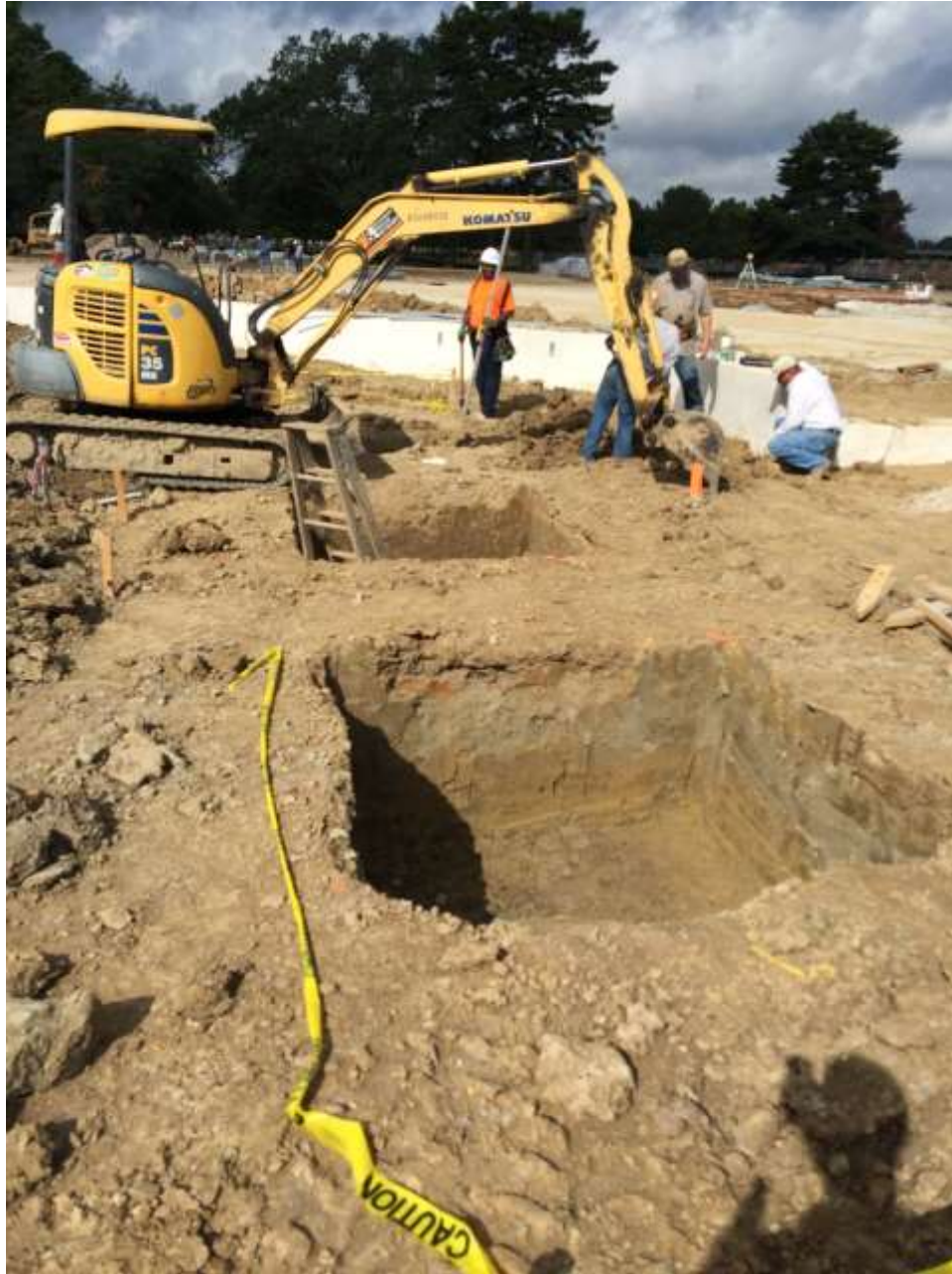
The flag pole foundations are being dug.
