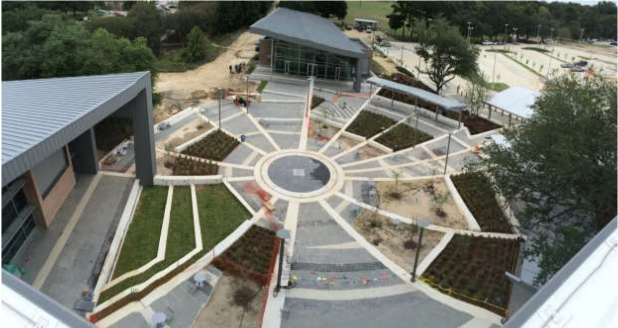
Looking from the roof to the Plaza.
