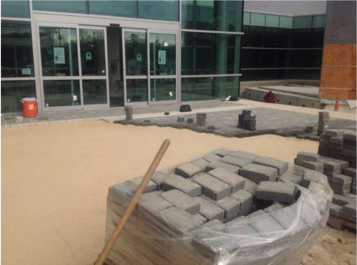
The pavers are being reinstalled at the Library Entry.
