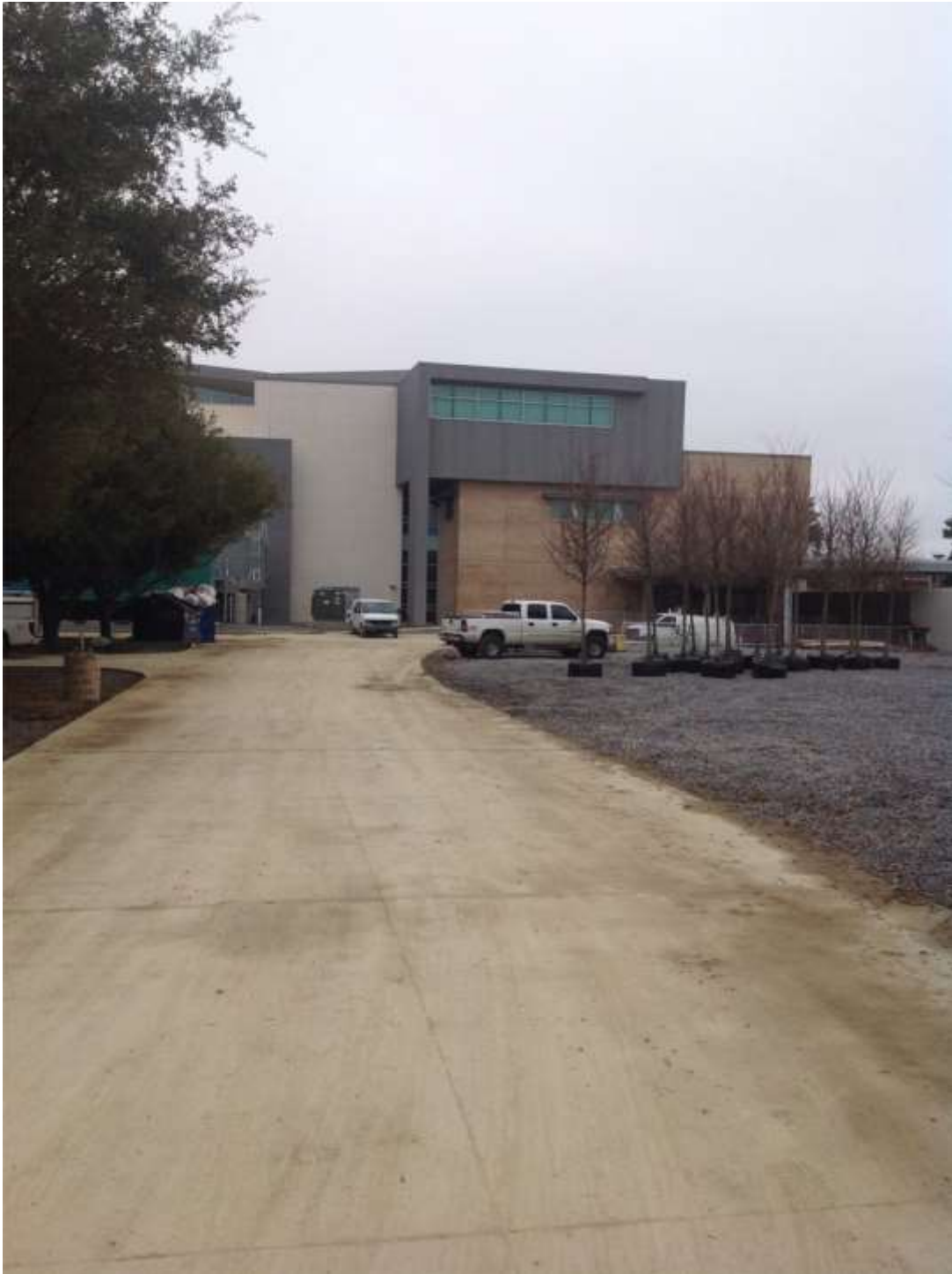
Looking into the Service Yard.
