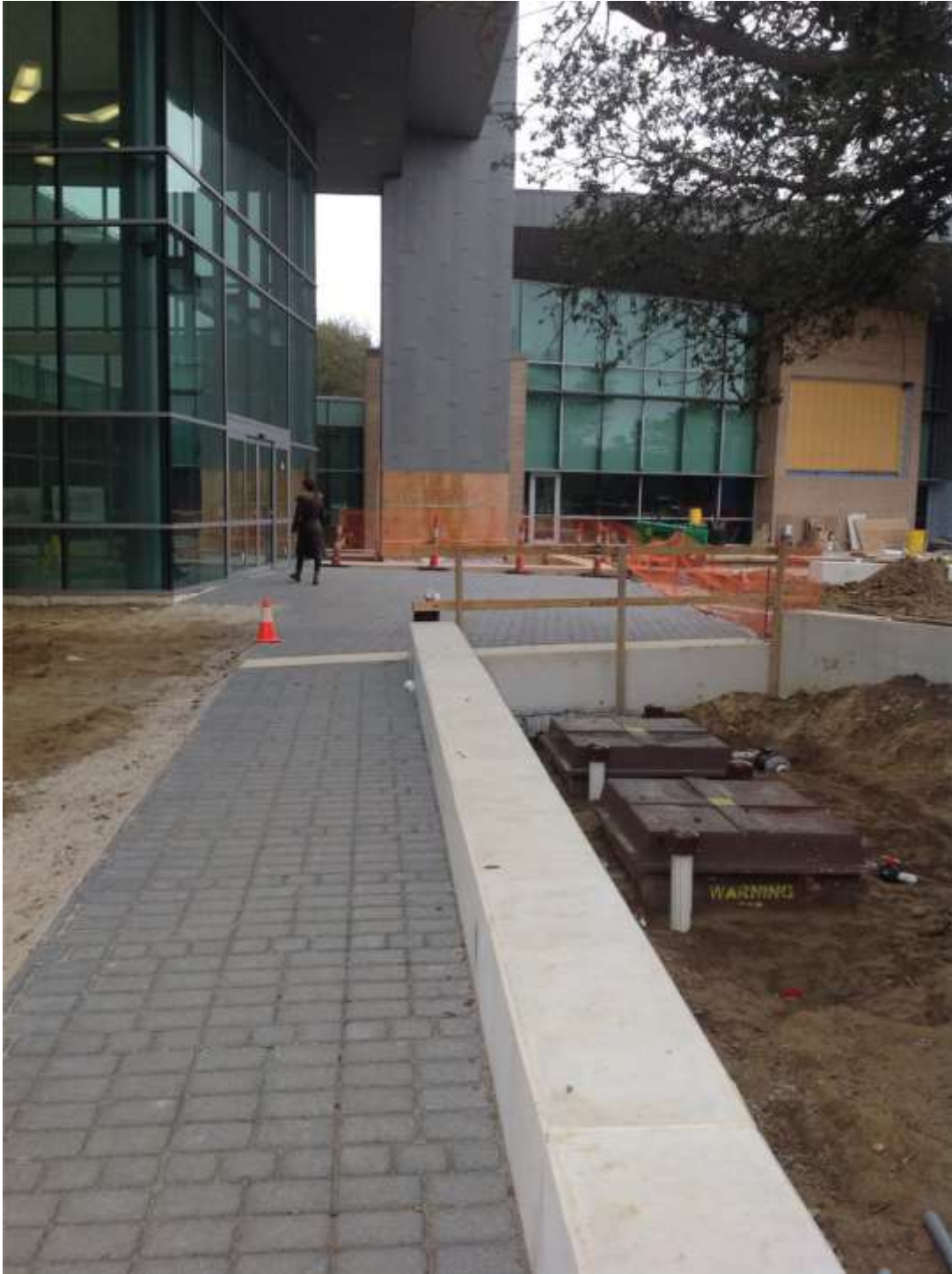
Looking toward the Library entry.
