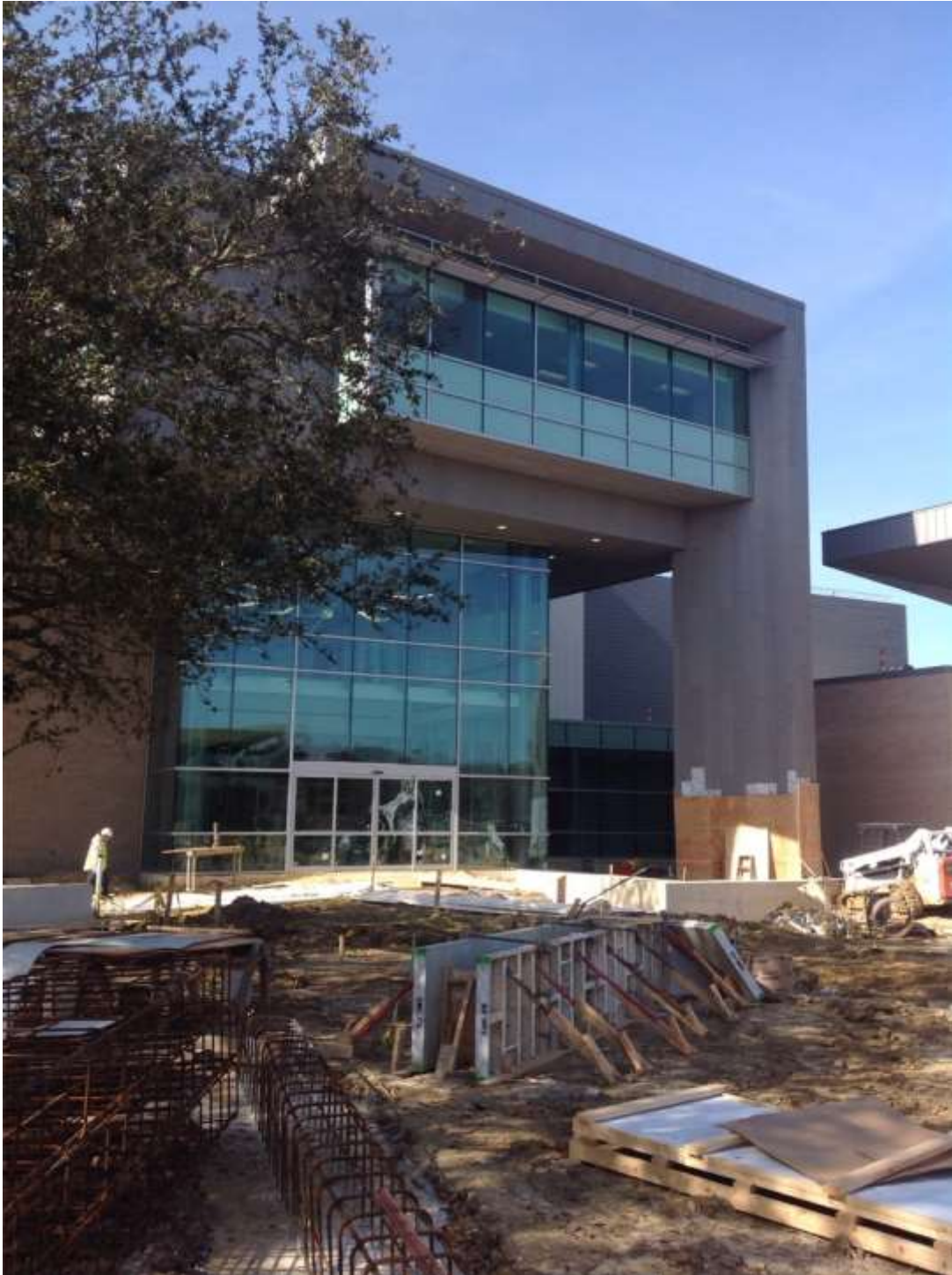
Looking toward the Library Main Entry from the Plaza.
