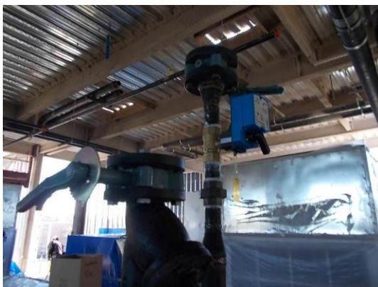
Protect open valve flanges
