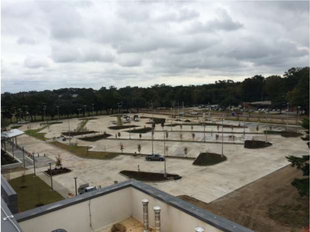
Looking from the southern roof garden to the new Goodwood parking area.
