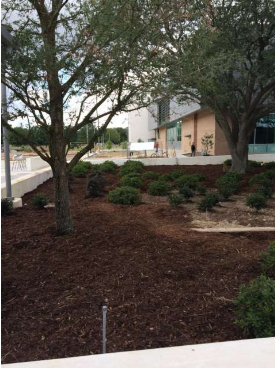
Looking at the bed preparation of the western planting area south of the Plaza.
