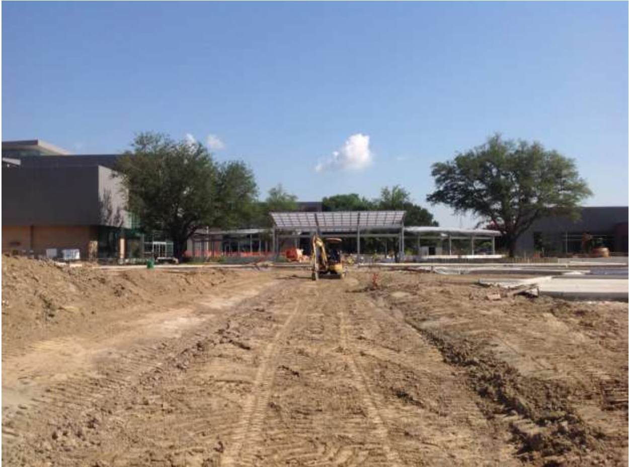
Looking from the parking lot to the Drop Off Canopy and the Plaza.
