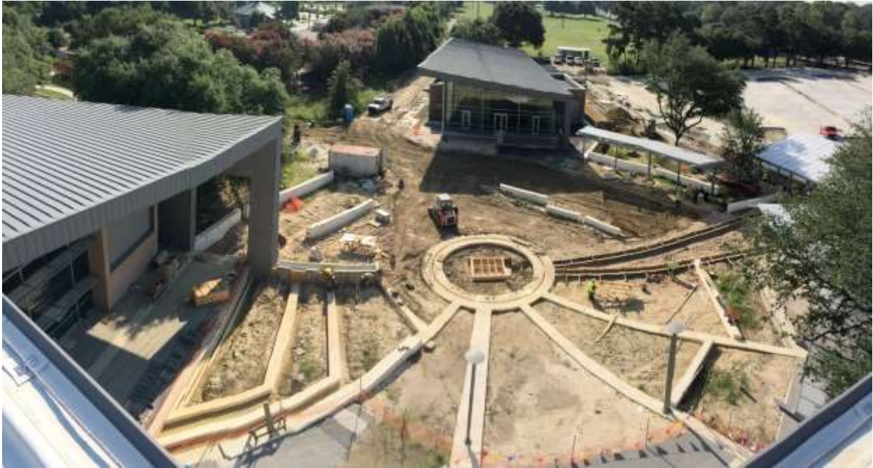
Looking from the roof to the Plaza.
