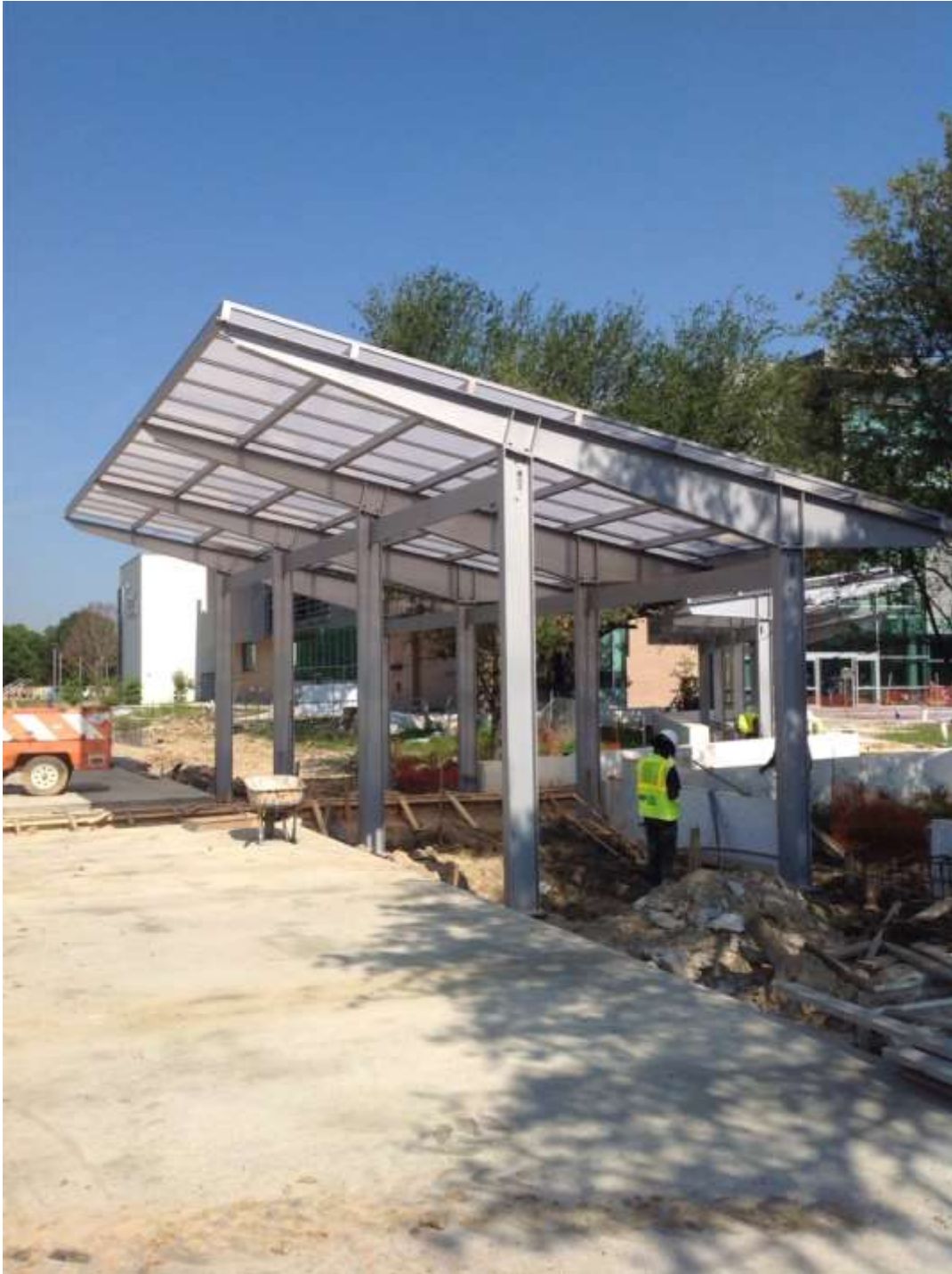
Looking west at drop off shade canopy in the parking lot.
