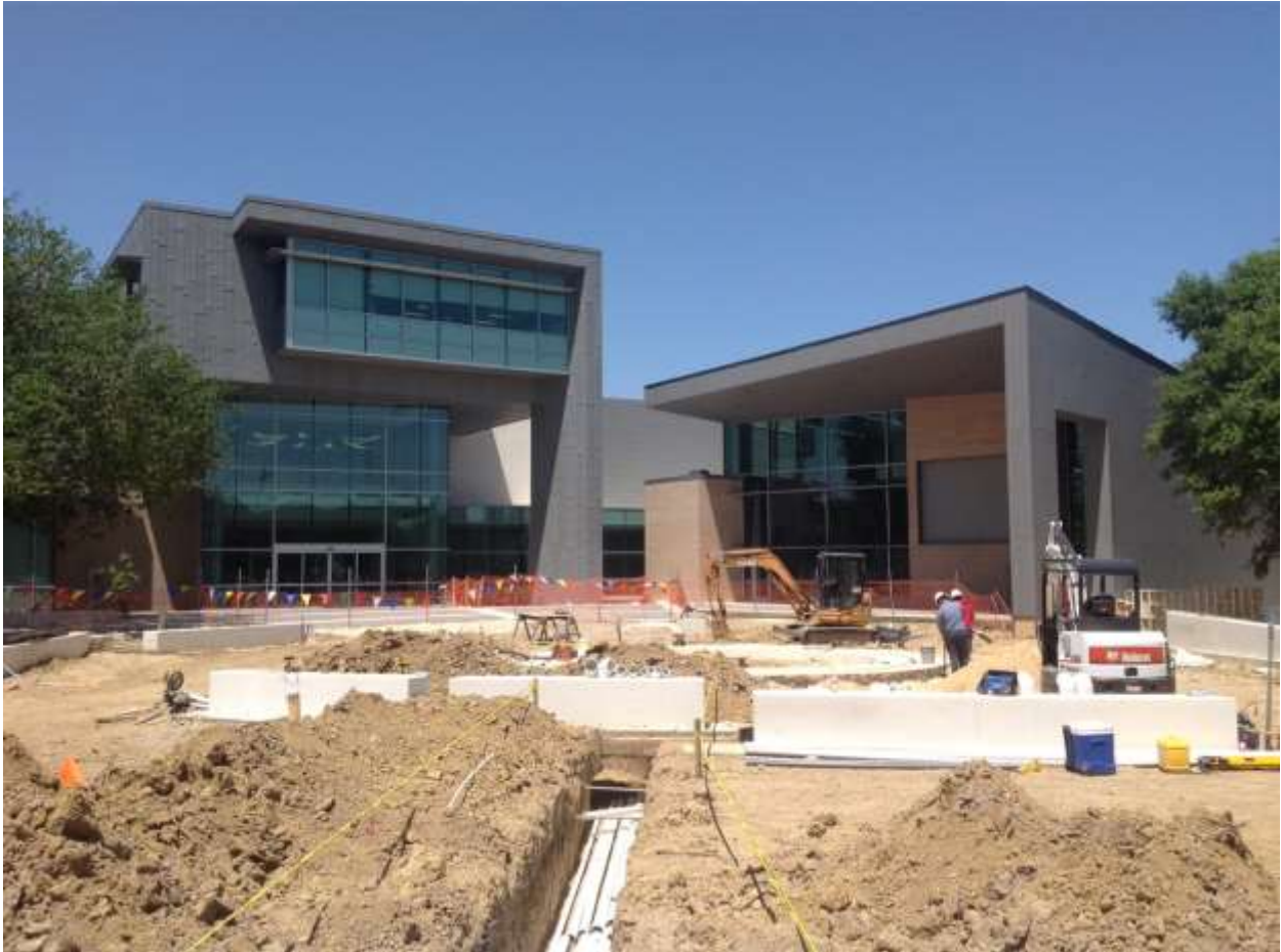
Looking Toward the Library's Main Entry.
