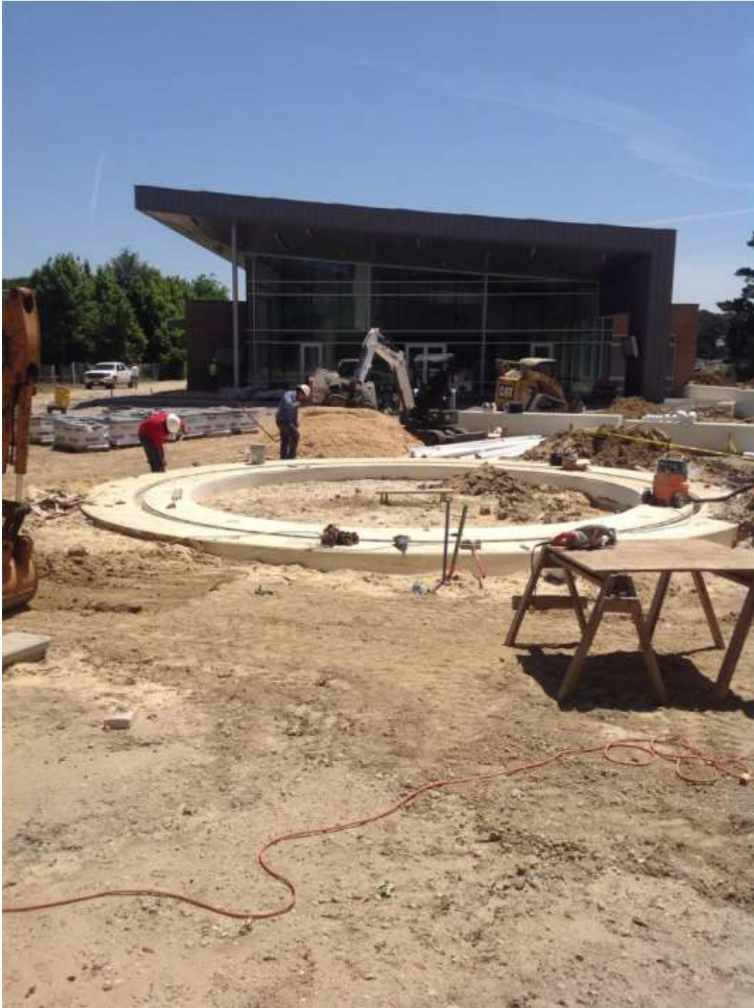
Looking east toward the Splash Pad.
