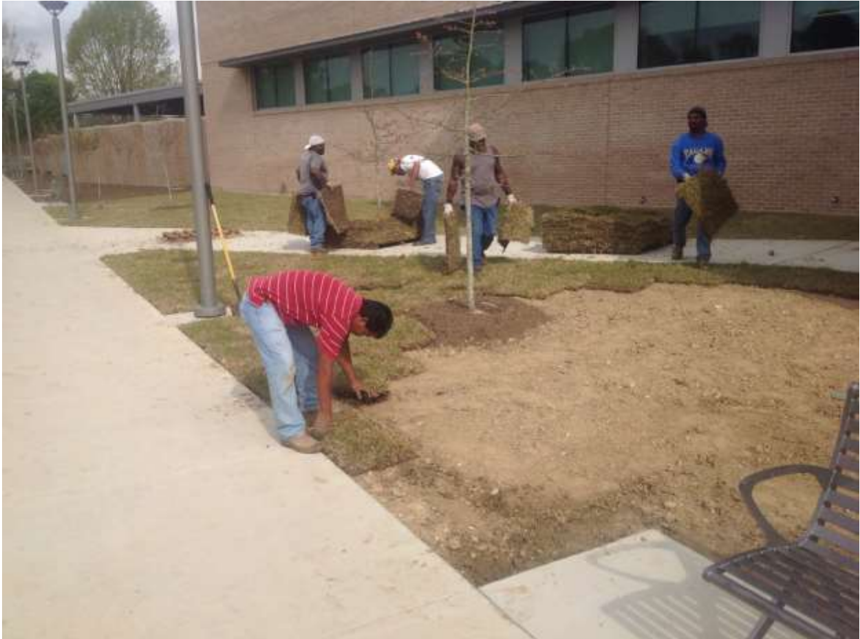
Sod is being installed.
