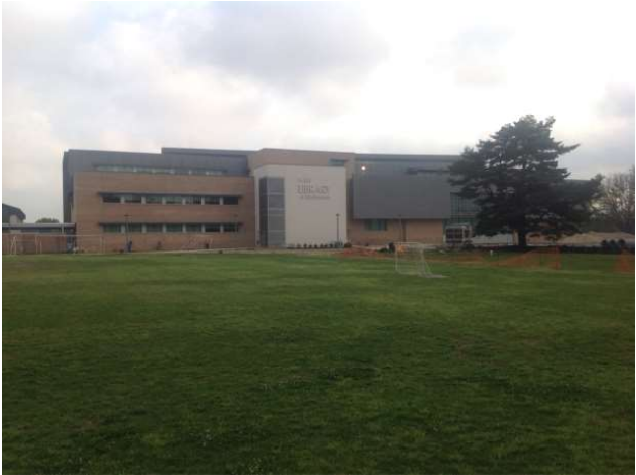
Looking toward the southern face of the library.
