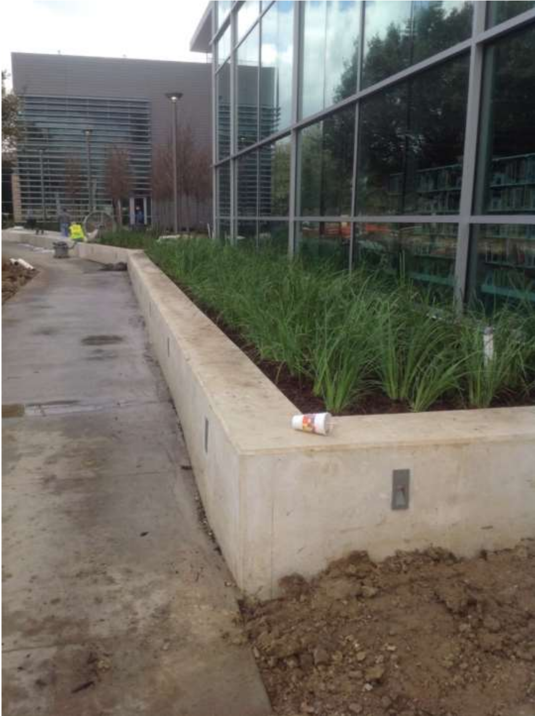
Looking toward the North Courtyard.
