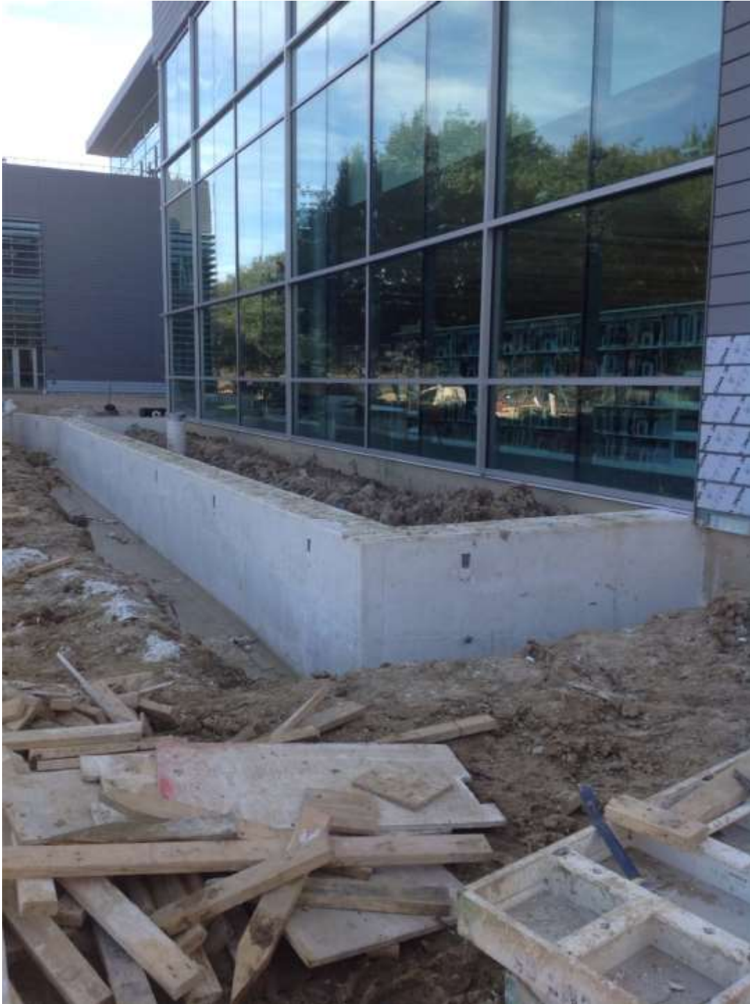
Looking toward the northern planters.
