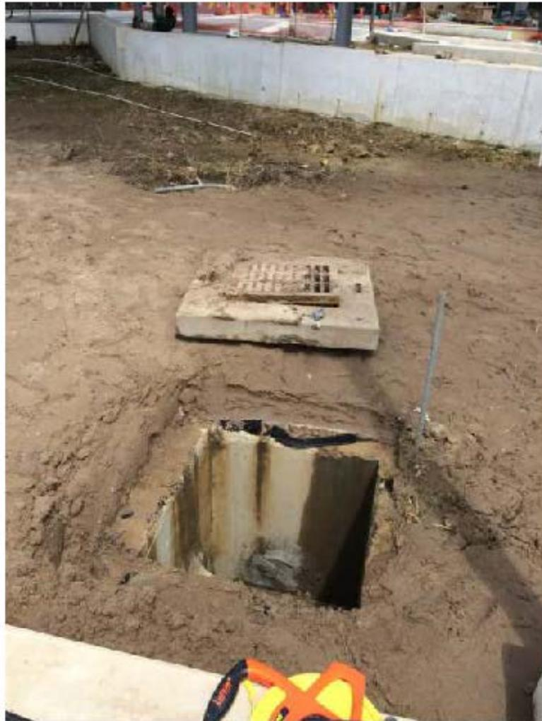
This catch basin is being lowered to ensure proper drainage.
